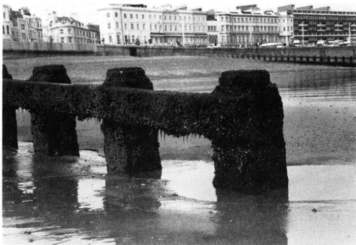
Fig. 3. Breakwater providing a solid surface for rocky shore molluscs – mussels, winkles and limpets.
