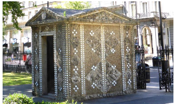
figure 1: The western shell hut.
