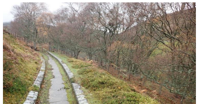
figure 4: The external surface of the culvert at Hopes Reservoir.
