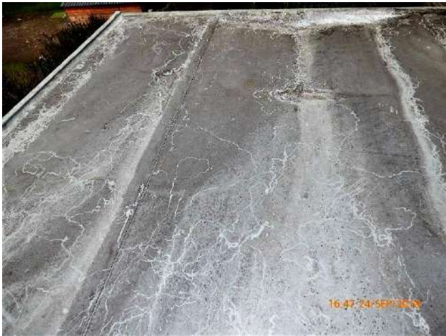
figure 1: View of the roof, showing how trails were concentrated in wetter parts.
