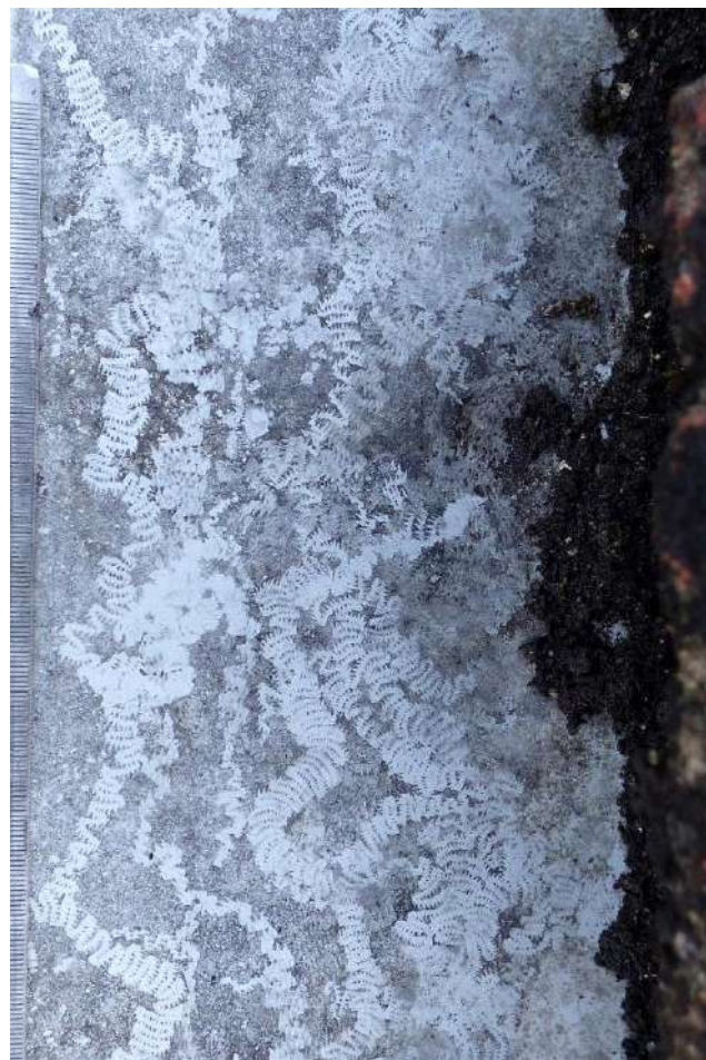
figure 6: Marks of intense feeding at the inner edge of the roof, where water accumulated.
