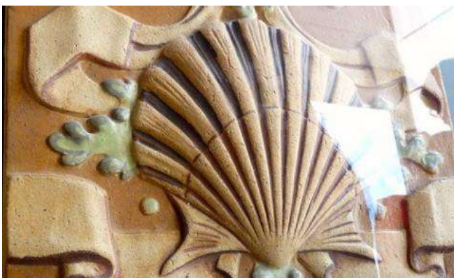
figure 2: A mould of the decorative ceramic Pecten shells that grace the exterior of Le MIM.
