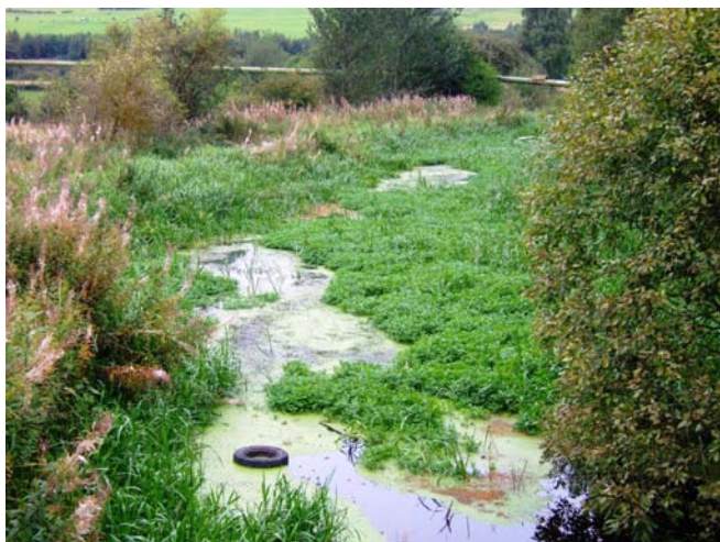
figure 2: The topmost section of the Monkland Canal, almost completely choked with vegetation.
