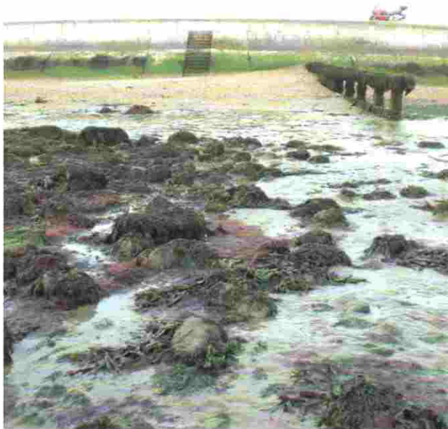
figure 2: Sea wall, groynes and boulders at Titchfield.
