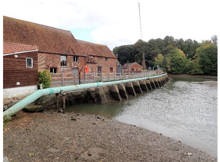
figure 2: Tide mill at Bartley Water near Eling, Southampton.
