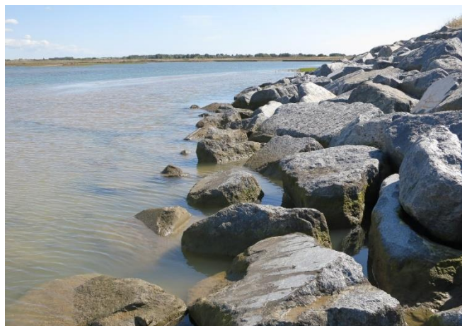
figure 22: Medmerry site B: rocky revetments at eastern entrance to Medmerry Reserve.
